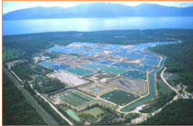
Some aquaculture ponds along the Great Barrier Reef coast are constructed in mangrove and saltmarsh habitats.
